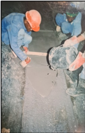
“Semi-self levelling” MicroConcrete being placed
