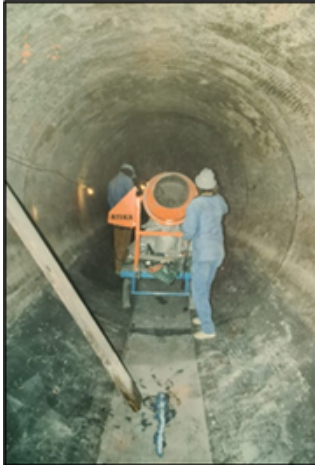
“Semi-self levelling” MicroConcrete being placed
