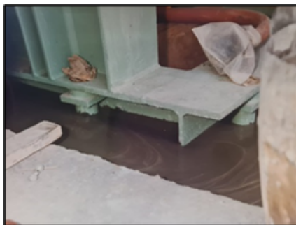
HS60 being pumped under large base plate
