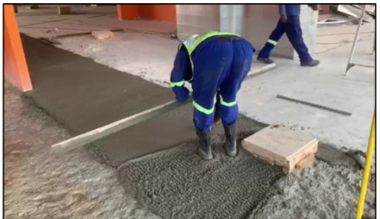
MicroConcrete repair to industrial floor
