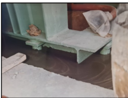
HS60 being pumped under large base plate
