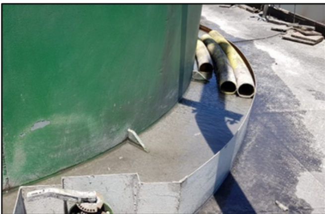
MicroConcrete placed by tremie
