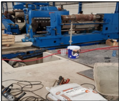
MS40 being pumped under a machine
