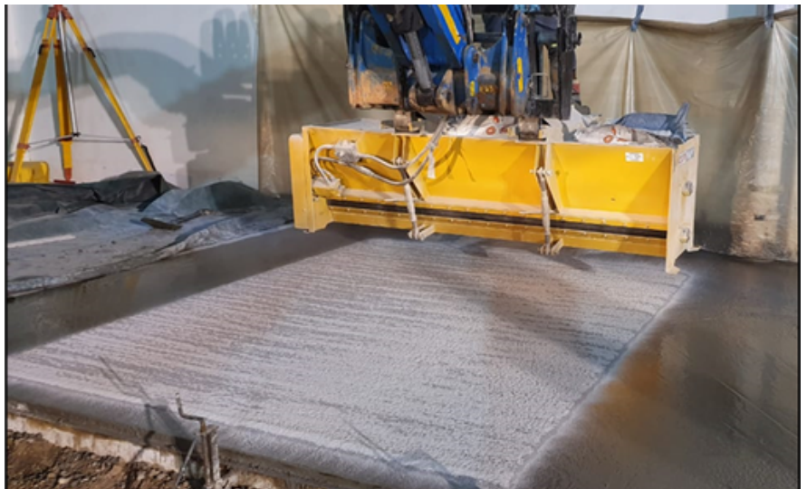
MBFT dry-shake may be manually or mechanically applied, dependent on the Contractor's equipment
