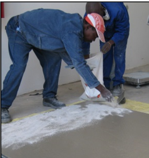
MBFT dry-shake may be manually or mechanically applied, dependent on the Contractor's equipment
