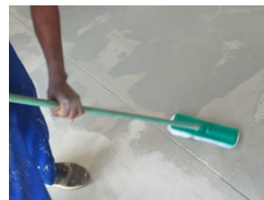
Fibre pad application
