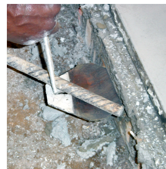
Dowel removal for shutter stripping
