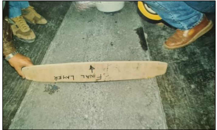
Simple device used for “Armco” profiling
