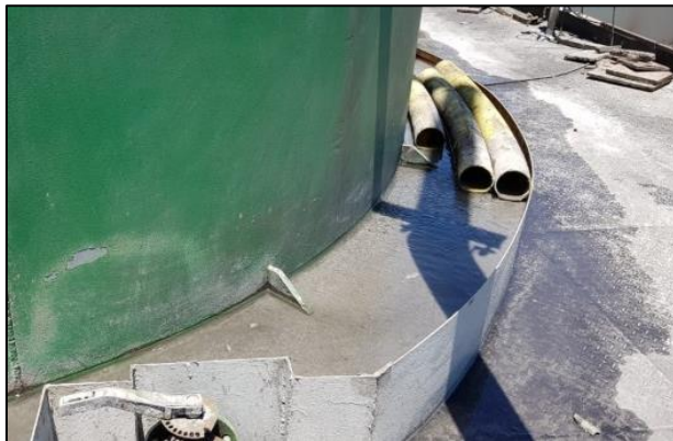
MicroConcrete placed by tremie
