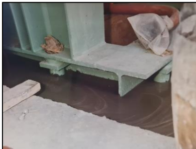
HS60 being pumped under large base plate
