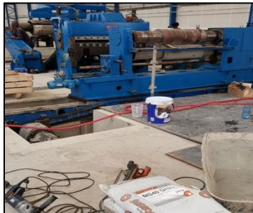
MS40 being pumped under a machine
