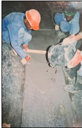
“Semi-self levelling” MicroConcrete being placed
