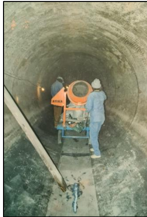
“Semi-self levelling” MicroConcrete being placed
