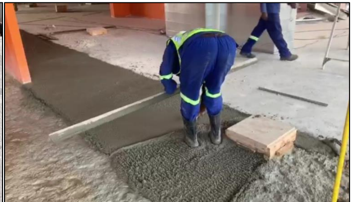
MicroConcrete repair to industrial floor
