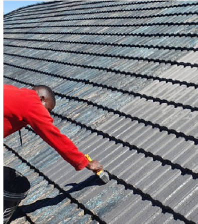
Apply the Roof RENEW
