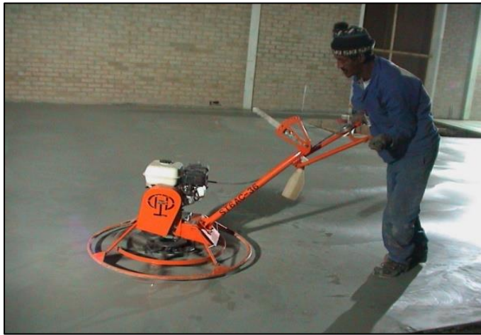
6-blade Powerfloat for finishing MBFT floors
