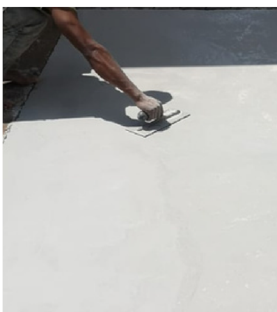
Apply the coating
