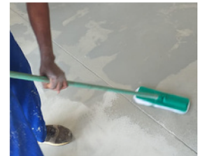
Fibre pad application
